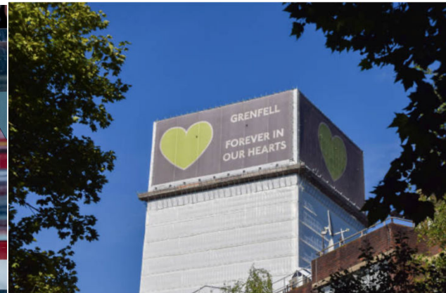
Further system failure...?
